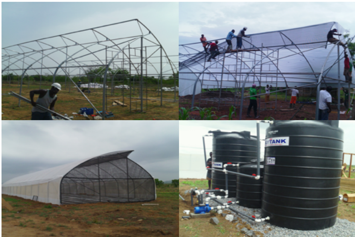
Figure 14: Greenhouse Construction at Akuse
